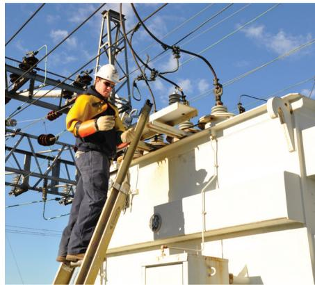
*Lineman Apprentice Alex Aydlett replaces arrestors on the Edenton Substation, while it was de-energized.*
