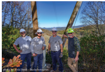
From left are: Albemarle EMC Crew Leader Bobby Upton, Lineman Drake Trueblood, Lineman First Class Chris White and Alvey Lester, chief lineman for Northwestern Rural Electric Cooperative.
